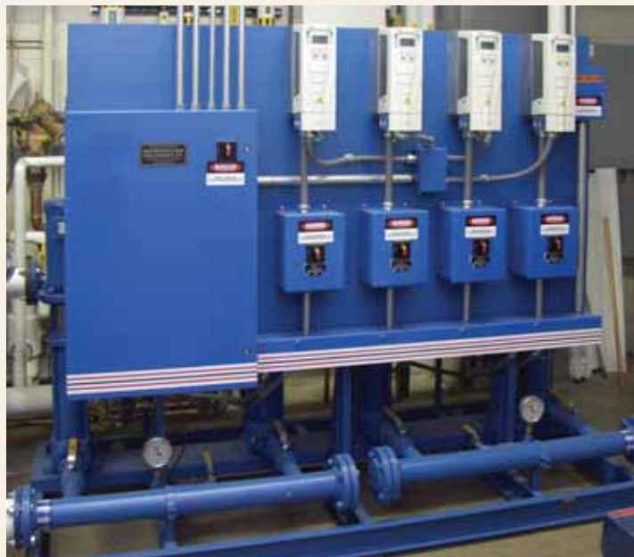
A Metropolitan Varipac System 2000 booster system, responsible for supplying separate pressures of hot and cold water during testing of various plumbing fixtures such as flush valves, shower valves, spray valves and sink fittings.
