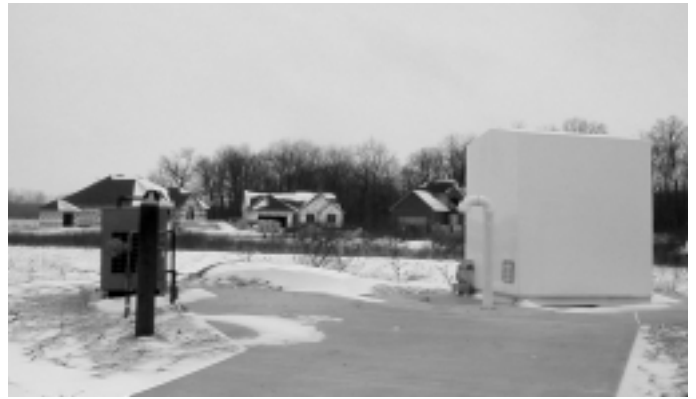
A recently installed walk-in housed valve station located in Monroe, Mich., 30 miles south of Detroit. Monroe is experiencing unprecedented growth, which required them to install new sewage lift stations near the new housing developments.
