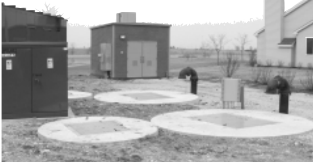
The completed lift station site in Romeoville.
