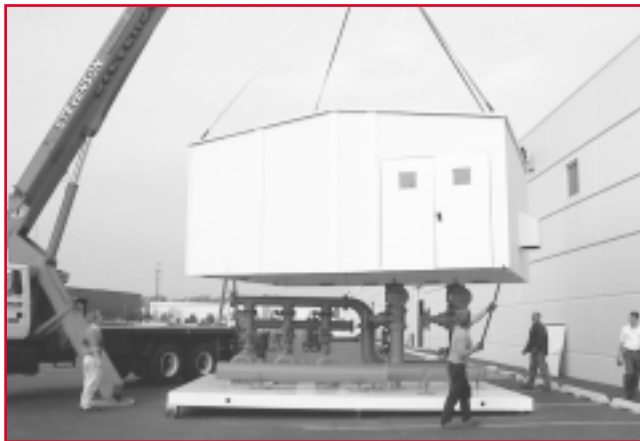
The modular enclosure being raised and set atop the steel frame.
