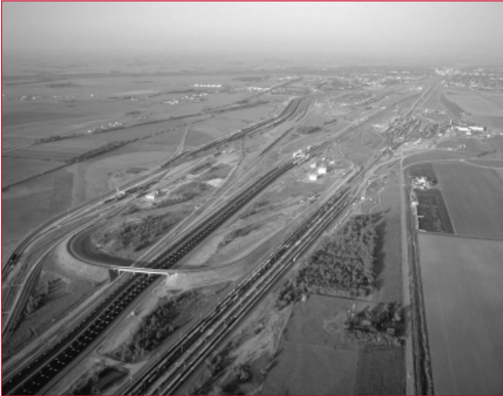
Pictured is Union Pacific Bailey Yard, the nation's busiest train yard located in North Platte, Nebraska. Metropolitan Industries raced against time in order to complete the installation of a prefabricated sewage pump station.
