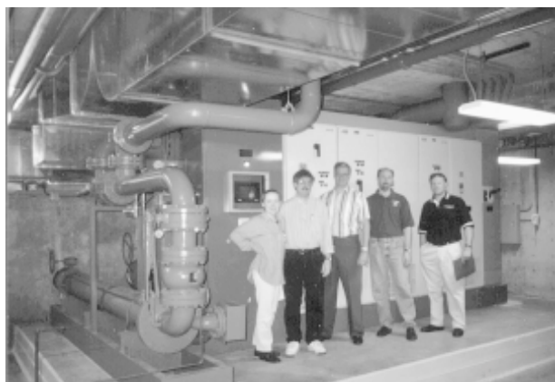
Left to right: Debbie Zentmyer, local Communications Asst. U.L.; Ken Cutler, Chief Plumbing Engineer; Larry Gesiakowski, V.P. WMA Associates; Ray Komorowski, Fire Protection Engineer; Mark Brickey, Metropolitan Pump
